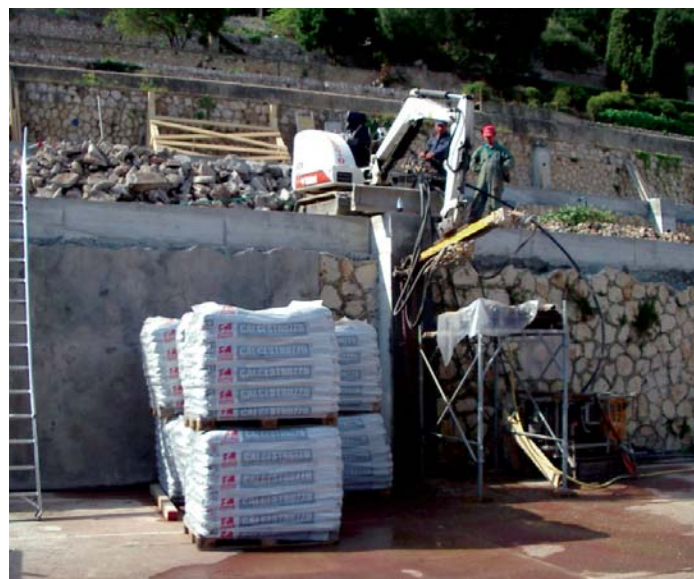
Terracing made with retaining walls reinforced in structural CALCESTRUZZO FIBRATO .
