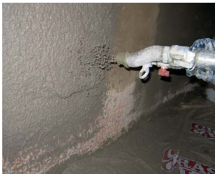
MALTA BASTARDA FIBRORINFORZATA can be applied by hand or pumped with a suitable pump (Type Step 120 from Imer International).
